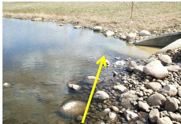
Sediment falls out immediately
