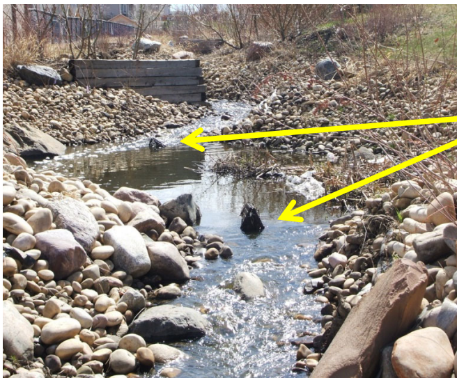
Clearflow Gel Flocculant™ Blocks placed in the feed stream to the ponds
