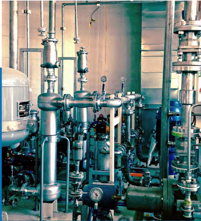
FIGURE 1: GDT Ozone Contacting Skids at Buckingham WTP
