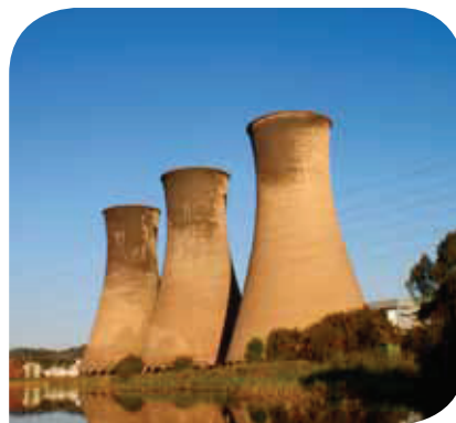
Example of cooling towers
