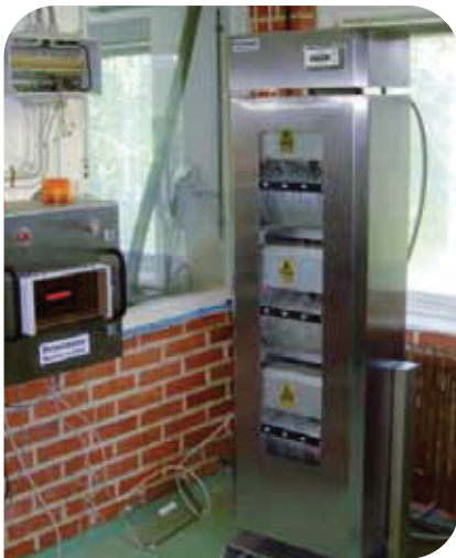
Ljungskile WTP during installation of the Primozone GM18.
